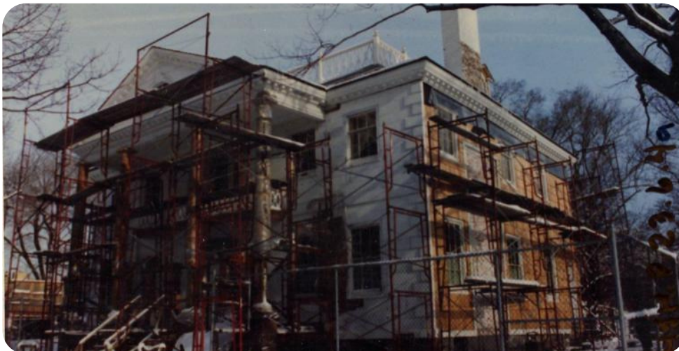
During the 1990 restoration
